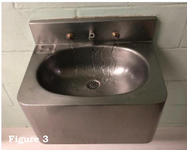
Figures 3 and 4. Leaking Sink (left) and Toilet (right) Observed in Folkston IPC Housing Units Where Detainees Were Held
