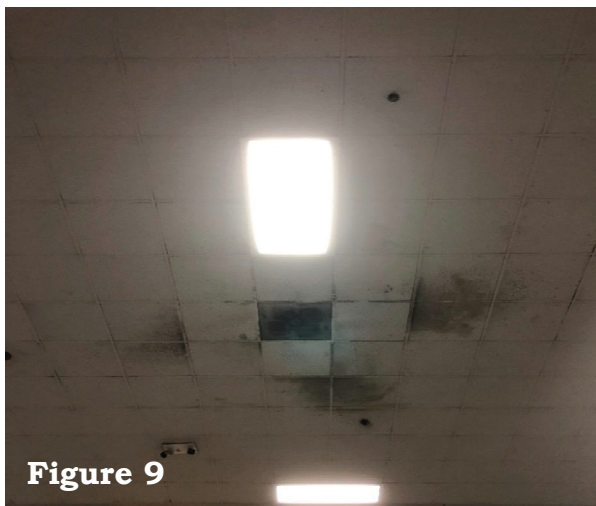
Figures 9 and 10. Ceiling Observed in a Folkston IPC Detainee Housing Unit, Showing Water Damage and Mold on the Ceiling (left) and in the Vent (right)
