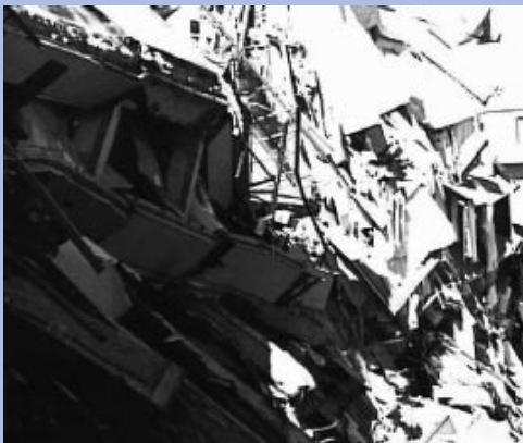
The New Orleans Riverwalk suffered extensive damage when it was struck by a bulk carrier vessel in 1996.
