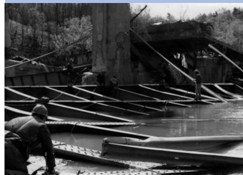
Ten people died when a New York State Thruway bridge collapsed in 1987. This was one of several NTSB-investigated accidents that resulted in improved underwater inspections of bridges and their footings.
