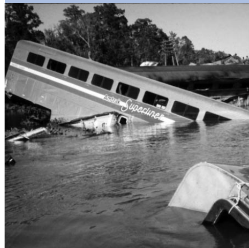
Forty-seven lives were lost when an passenger train derailed on a bridge and plunged into a bayou in 1993. Barges had previously hit the railroad bridge displacing the track.
