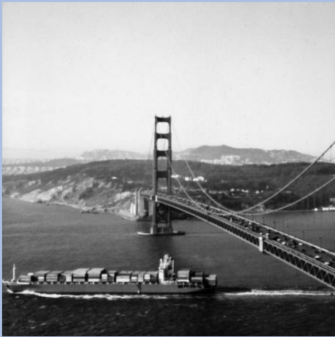
Voyage data recorders are now required on ships like this one in San Francisco Bay.
