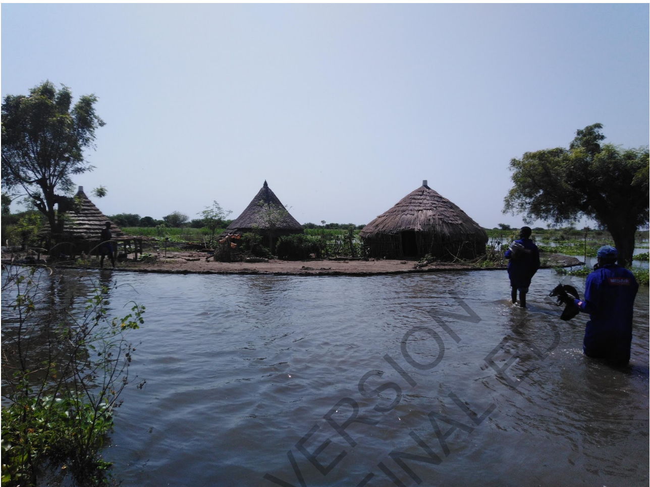
Figure Box 9.2.1: Indigenous earth walls ( hayit ) built by indigenous people in Akobo, Jonglei Region, South Sudan to protect their houses/ infrastructure from the worst flood in 25 years occurred in 2019. The wall is 1–2 m high. Photo credit, Laurent-Charles Levesque .
