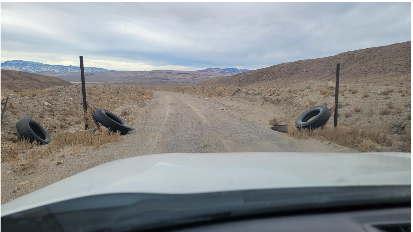
Figure X23: Cattle grate west of Rhyolite Ridge on Cave Springs Road filled in with sediment and passable to cows.
