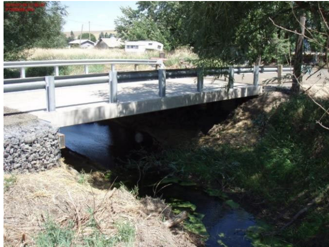
FIGURE 2 Thornton Depot concrete bridge.
