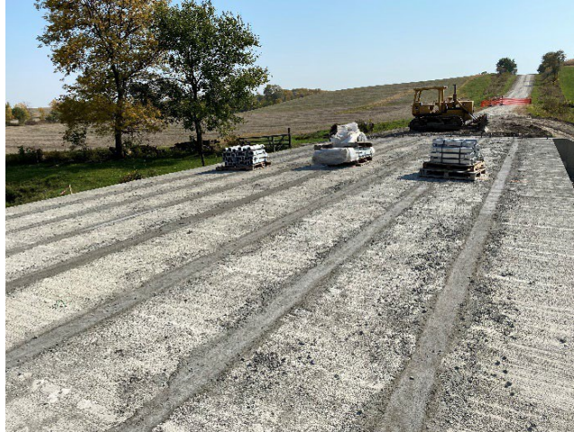
FIGURE 8 Bridge inspection results.
