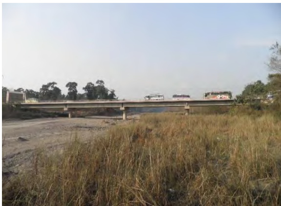
FIGURE 1 Photo and figure of major bridges with a dry floodplain terrace that is ideal for wildlife movement through the bridge.
