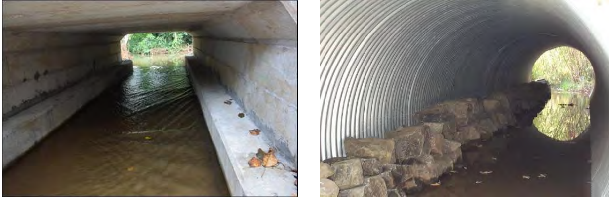
FIGURE 3 Culverts with a raised bench constructed of concrete or retrofit with rock to provide a dry platform for wildlife movement through the culvert. (Photos from Adolfo Artavia and Randall Reeves).
