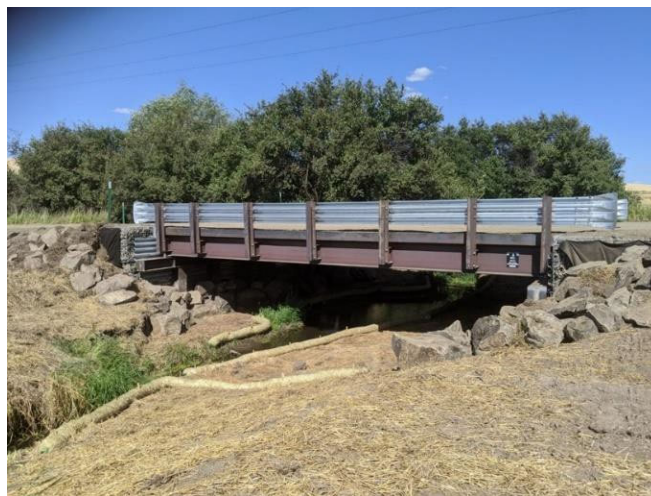
FIGURE 1 Seltice-Warner steel bridge.
