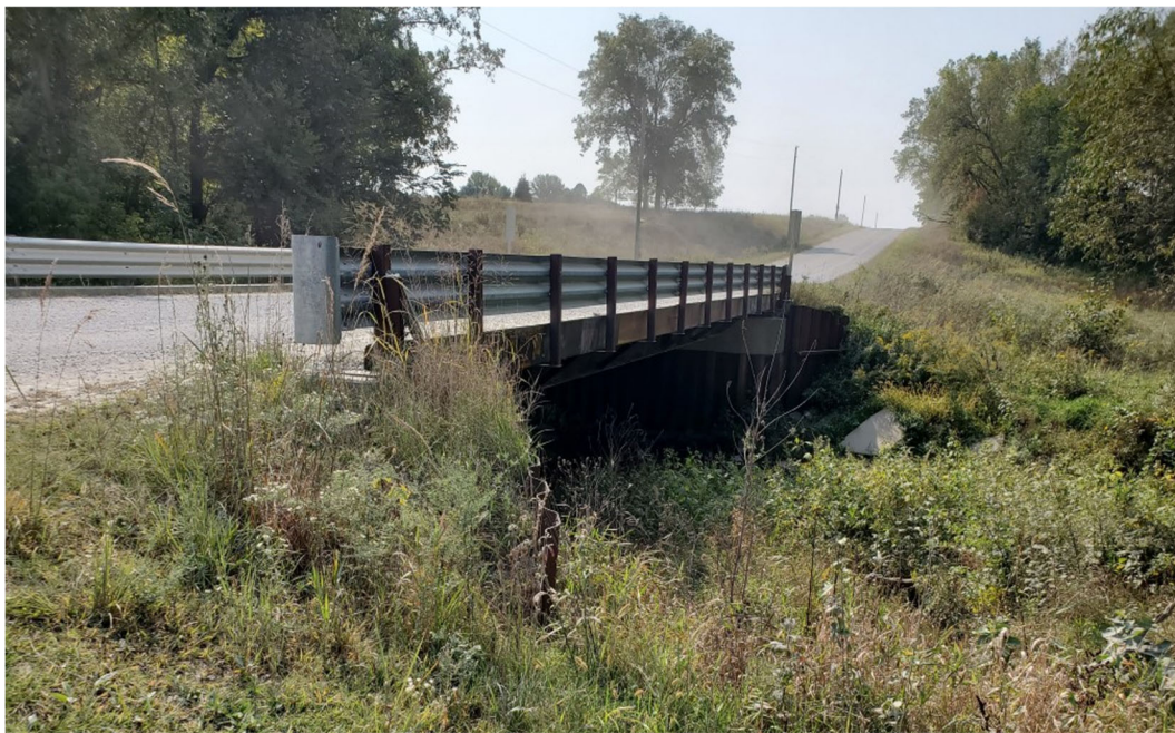
FIGURE 2 Typical 65-ft railroad flatcar bridge.
