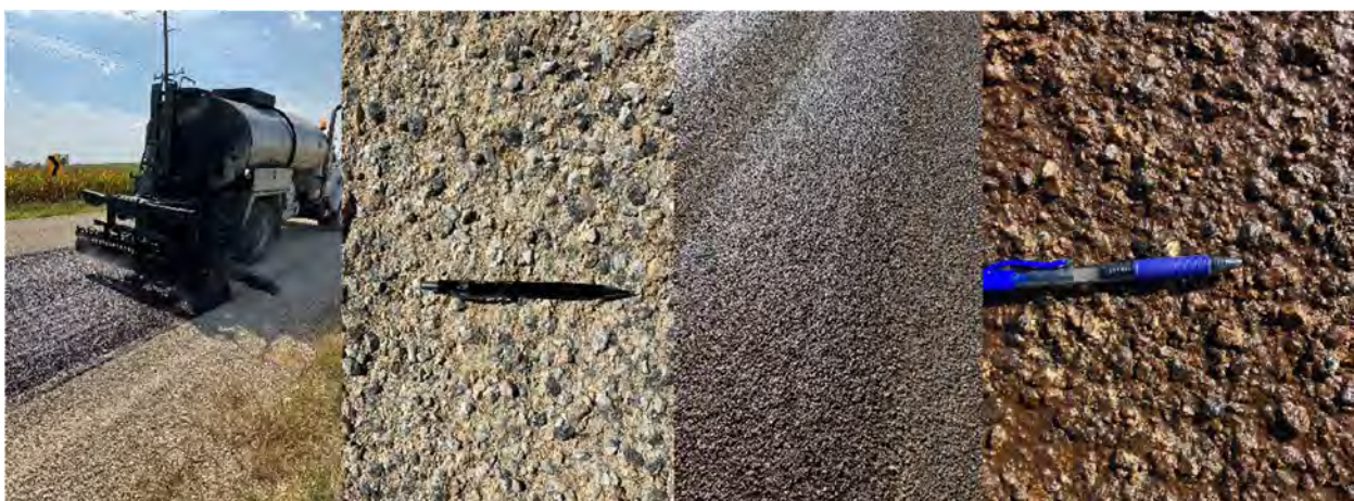
FIGURE 2 Cape seal construction. Photo by Clinton County.
