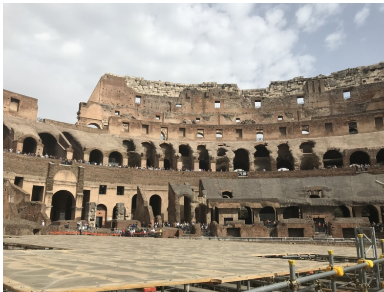
6.50 Interior of the Coliseum 2019. xiii
