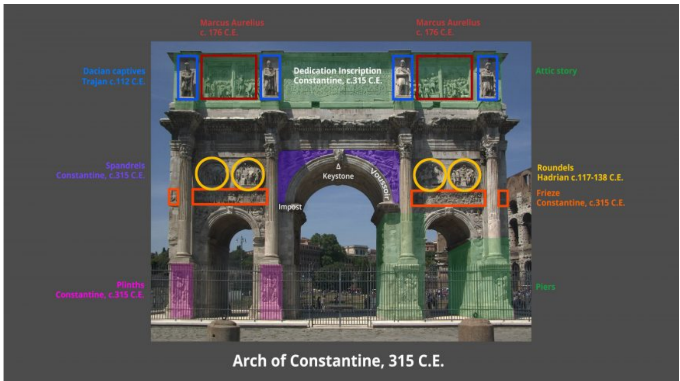
7.30 Diagram of the Arch of Constantine showing architectural features and spolia. 312-315 CE, Rome, Italy. viii
