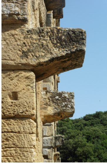
6.39 Stone projections at the Pont du Gard made for scaffolding ii
