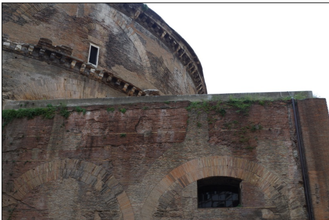
6.54 Exterior walls of the Pantheon. xvii
