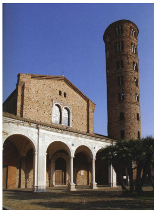
8.30 Marble portico of Sant' Apollinare Nuovo, which was rebuilt after the First World War. The entrance is on the west side of the church. vii
