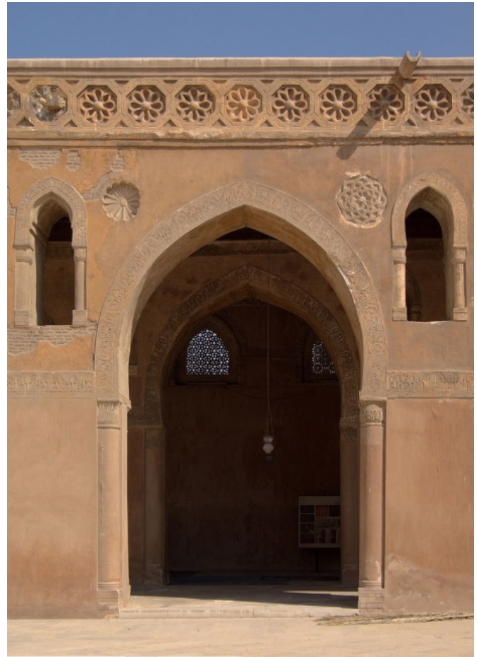
9.21 Mosque of Ibn Tulun, Entrance door. x
