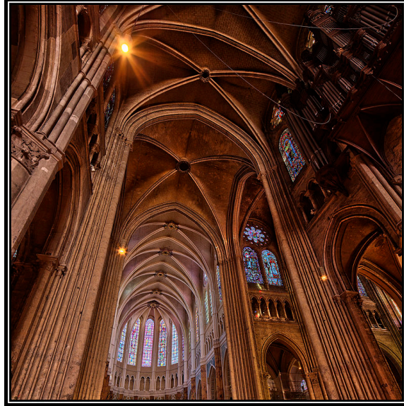
11.27 Chartres ribbed vaults in the nave. xi
