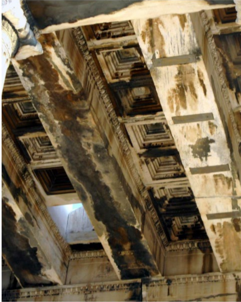
4.86 Coffered ceiling of the North porch of The Erechtheum , 421-405 BCE., Acropolis, Athens. xi
