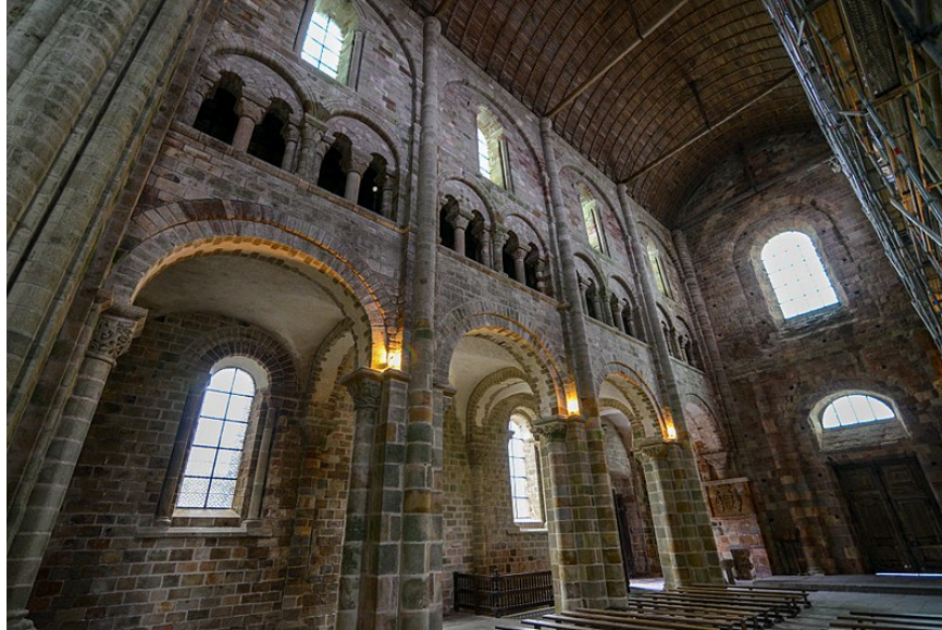
11.13 Abbey Church of Mont St. Michel has rounded arches, heavy support columns and tiny windows. xiv
