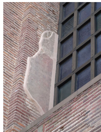
7.56 Remnants of the original plaster may be seen around the windows of the Throne Room. vi
