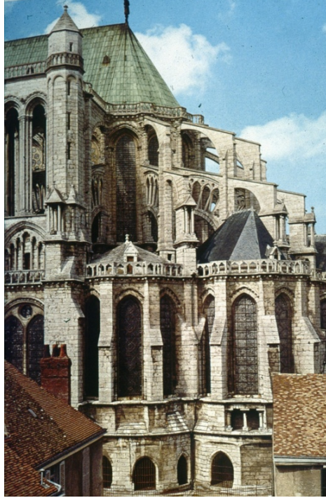
11.44 Flying buttresses of the choir at the east end of the cathedral of Chartres. xxix
