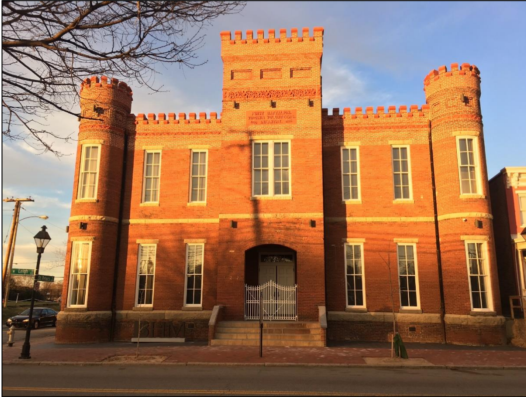
Figure 9. Leigh Street Armory, March 2016. Source: Historic Richmond.
