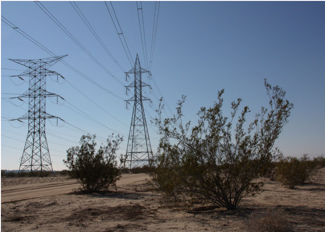
Transmission line on public lands in California, source: BLM
