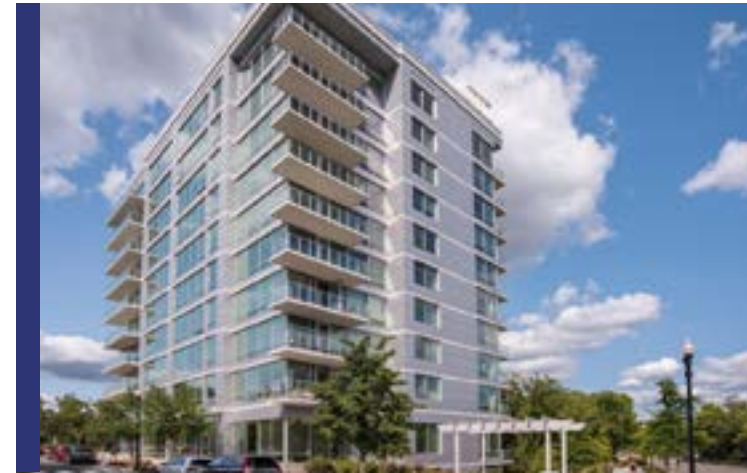
Verde Point - 11 CAF units in North Highlands (Source: AECOM)
