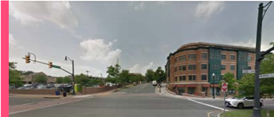
C-O-1.0: Mixed-use Building on 2101 North Monroe Street (Maywood)
