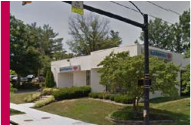
C-O: Bank on Lee Highway West of N. George Mason Drive (Leeway Overlee)
