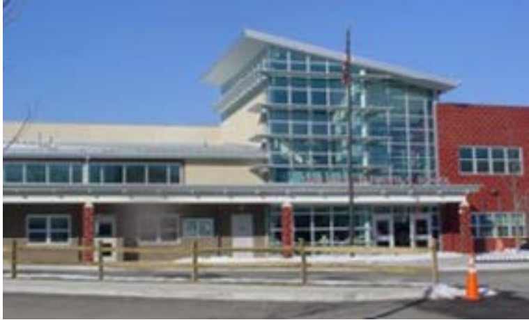
Glebe Elementary School (Source: APS)
