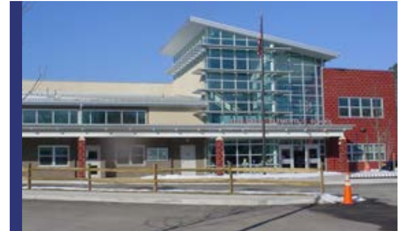
Glebe Elementary School (Source: APS)
