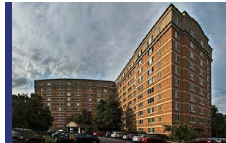
Potomac Towers - 324 MARKS units at 80% in HCD in North Highlands (Source: AECOM)
