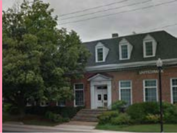
C-O-1.0: Bank and Office on Lee Highway (Leeway Overlee)
