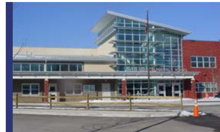
Glebe Elementary School (Source: APS)
