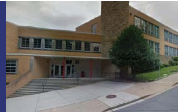
Stratford Junior High School (Source: AECOM)
