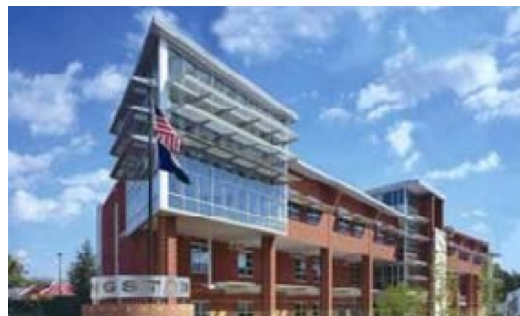
Langston Brown Community Center (Source: APS)
