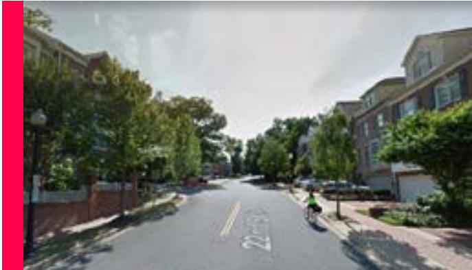
C-O-1.5: Townhomes on 22nd Street North (N. Highlands)
