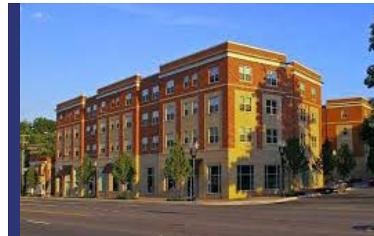
Hunters Park - 74 CAF units for seniors in Cherrydale (Source: AECOM)
